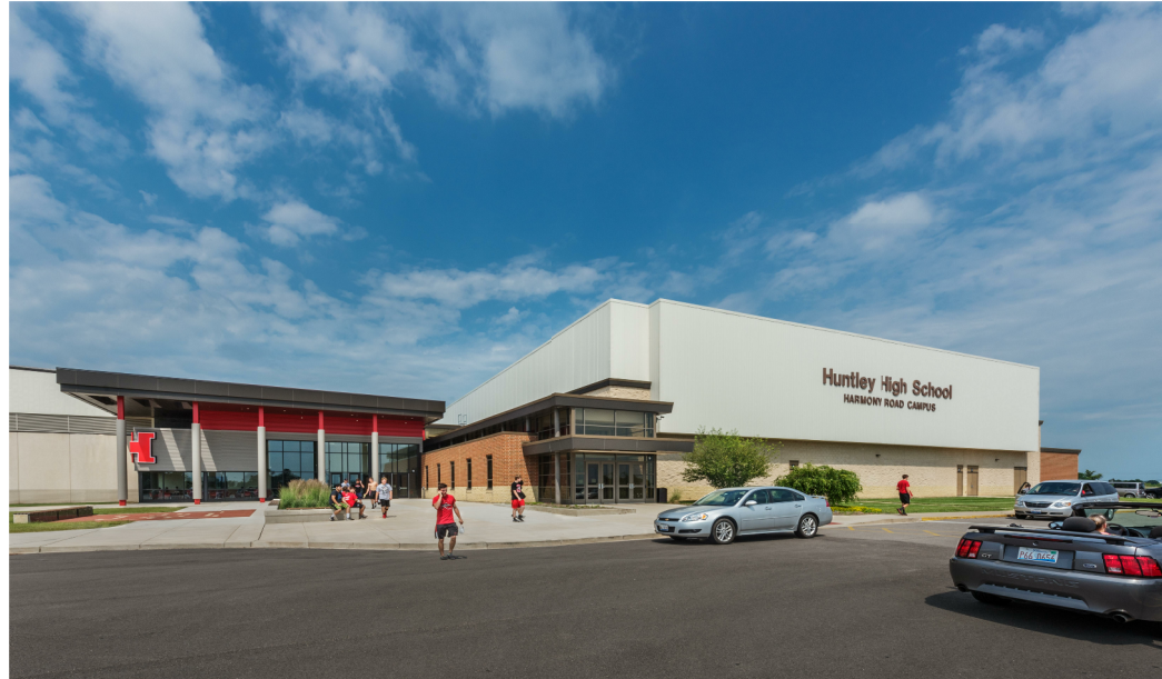
EXISTING THEATER ENTRANCE
